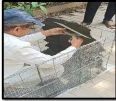
Fig 1 : Ferrocement work
