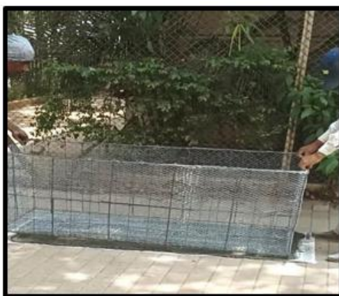
Fig 4: Base slab preparation
