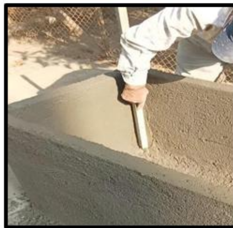
Fig 8: Levelling
