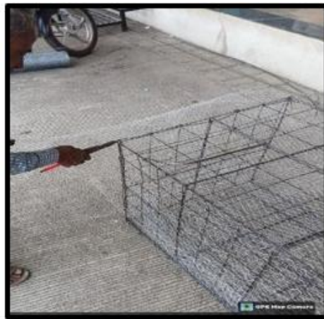
Fig 3: Applying G.I Chicken Mesh
